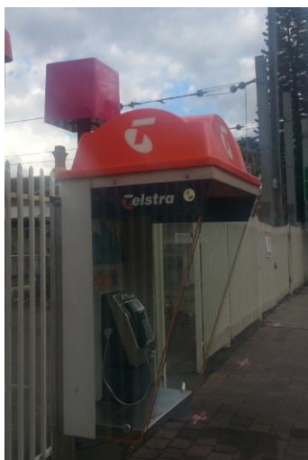
Public Telephone cabinet with Telstra Wi-Fi installation
