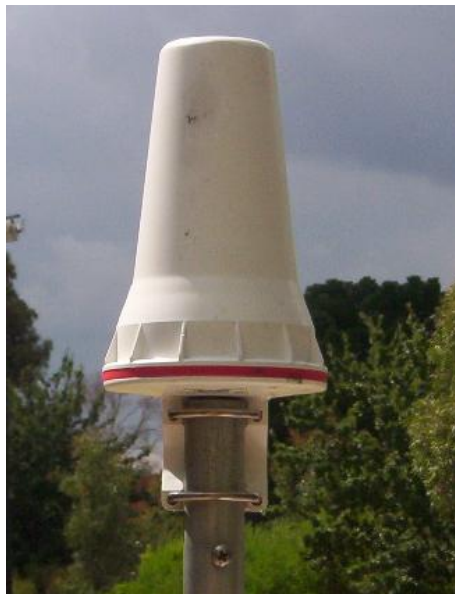
No EME Clearance Zone
