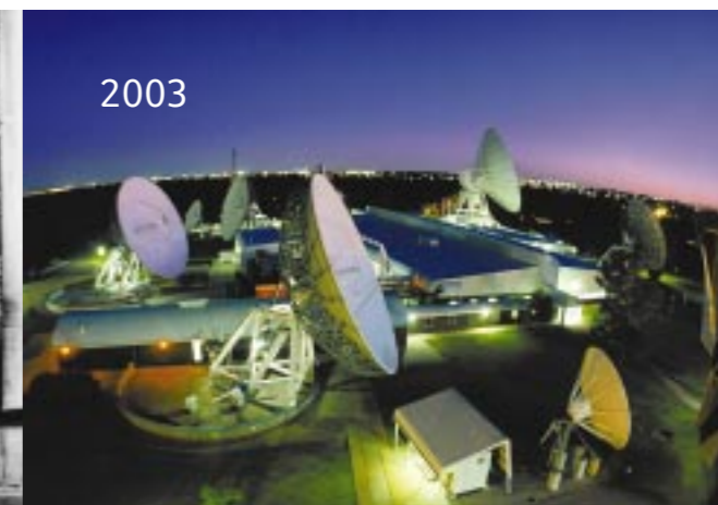
Satellite dishes, Gnamgarra Earth Station, WA.
