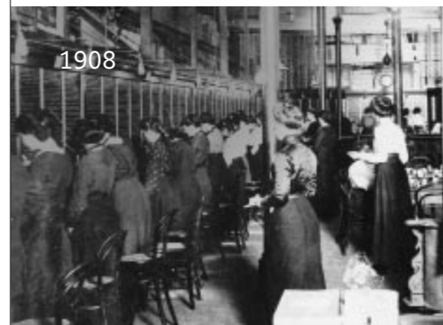
Telephone switchroom in PMG Exchange.
