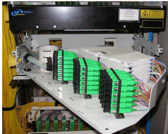
24 fibre COFTU panel
