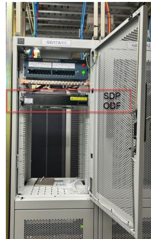
Internal – NBC Half Height Rack
