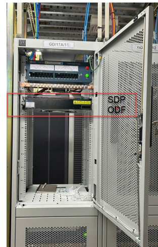
Internal – NBC Half Height Rack
