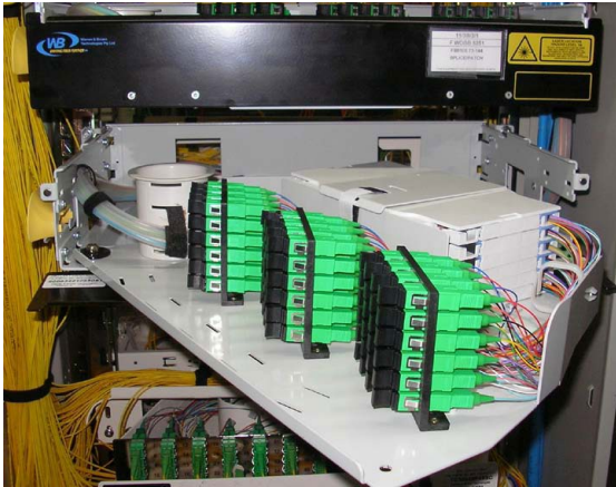
24 fibre COFTU panel
